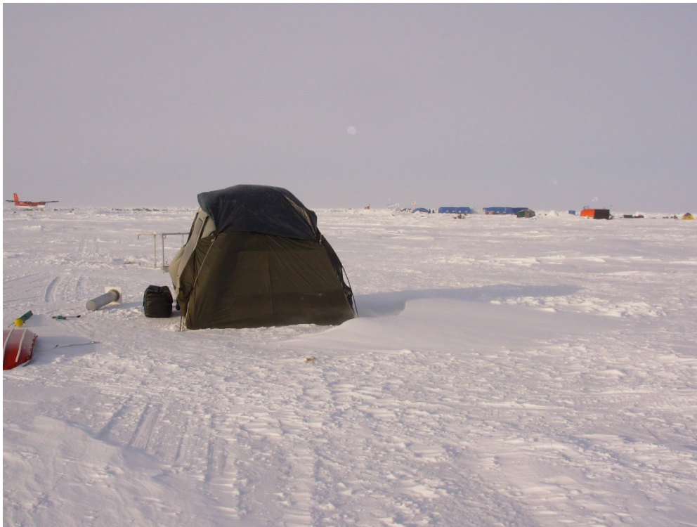
The installation site with working tent for the first half of the IBO (including IMB and Weatherex) on April 23, 2007. In the background are the tents making up ice camp Barneo and the Twin Otter aircraft parked on the runway.
