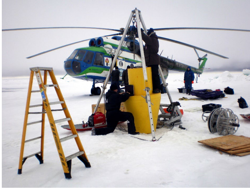
Immediately upon installation of ITP 26 (with conical supplemental flotation) the system's ability to transfer data from the underwater profile to surface package is tested. Kris Newhall performs the inductive modem test while Jeff Pietro begins disassembling the deployment apparatus. (Photo by Sergey Unovidov)
